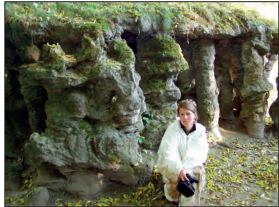
Figure 5: Fragment of the natural, sandstone colonnade at the entrance of Groty Mechowskie Cave with artificial column supporting concrete seal in the ceiling, situated directly to the right of the lady (photo J. Urban, 2005)
