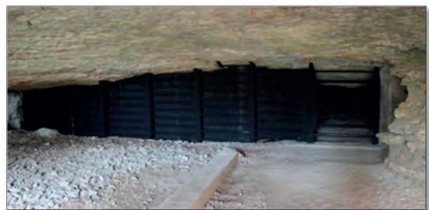
Illustration 2: Natural entrance: view of wooden panels (left) and the grid-door (right)
