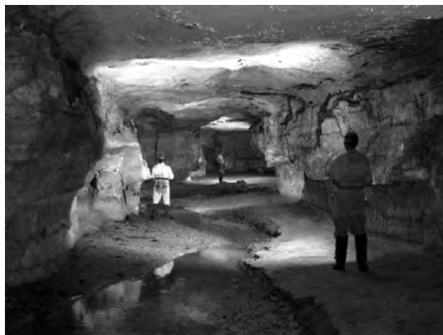
Figure 4. Double-roof channel. Photo by: J. A. Labegalini.
