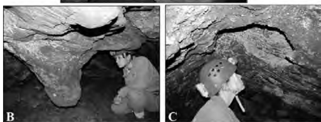
Figure 7. (A) Calibrated conduit with the presence of a crack between the itabirite and the detrital iron crust; (B) Pendant, relic form which indicates the coalescence of conduits related to a dissolution process; and (C) Ceiling dome formed at the top of the Gruta do Cascalhinho.
