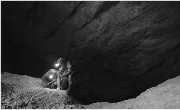
Figure 7. Cavern at km 1+415 in Biokovo tunnel.
