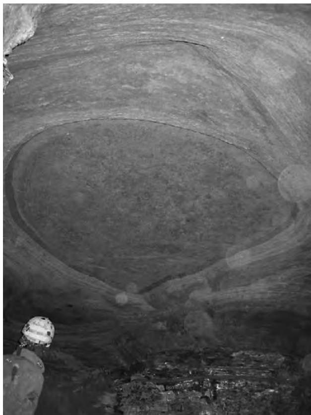
Figure 8. Slab detachment from the vault in lacustrine deposits of a lignite mine.
