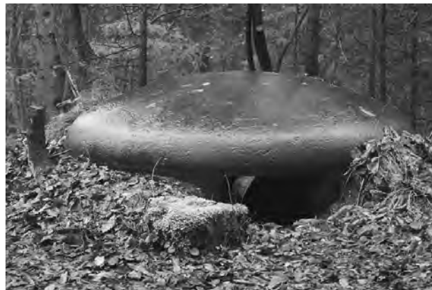
Figure 7. Steel cupola on top of the bunker. Below it, the northern portal of the tunnel is filled with rubble and hidden.
