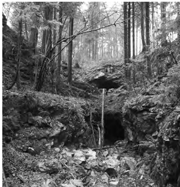
Figure 2. Southern entrance showing the pioneer tunnel (lower aperture) and crown (upper aperture).
