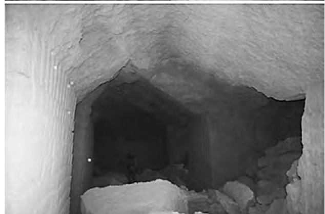
Figure 9. Double (above) and single (below) arches produced by failures at the vault.
