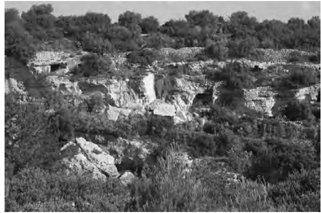
Figure 7. Rock failures in a gravina at Massafra (Apulia), threatening several artificial cavities.
