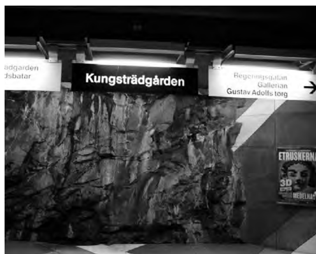
Figure 1. Kungsträdgårdens subway station, located more than 30 m below the surface in central Stockholm, Sweden. A large part of the wall is covered with the moss Eucladium verticillatum . There are also several distinct biofilms and speleothems.
