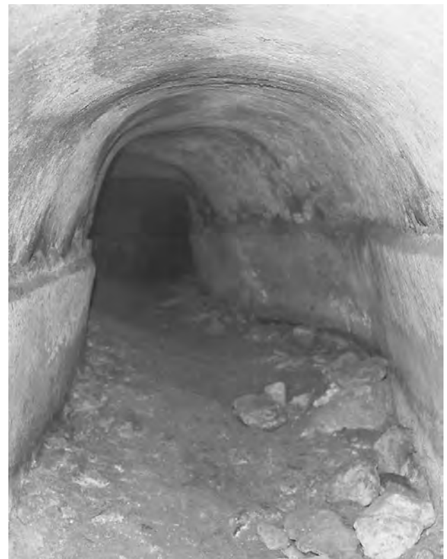
Figure 2. Crypta neapolitana : the aqueduct at a junction between two digging teams.
