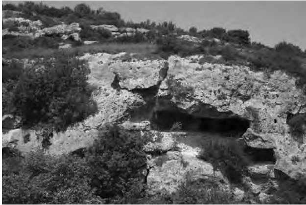
Figure 4. An artificial cavity in calcarenite rock, strongly controlled by a tectonic discontinuity.
