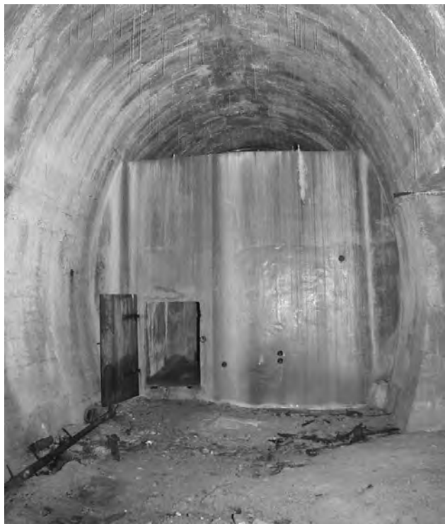
Figure 6. Bunker in the finished part of the tunnel.
