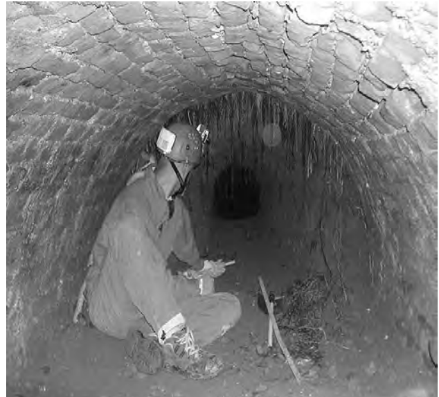
Figure 7. Bastione Verde tunnel at Torino (Italy). Photo: F. Milla.
