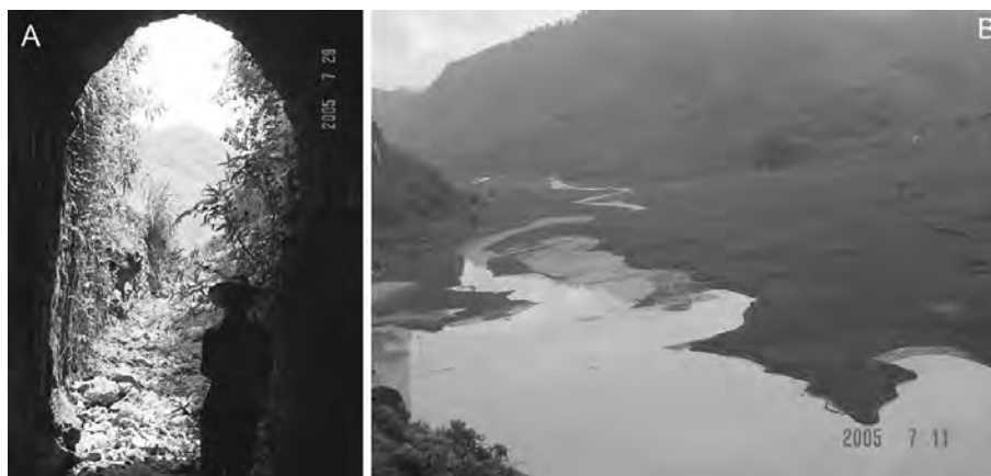
Figure 7. Flood in karst area and engineering for flood discharge, A: tunnel in the Dongni for discharge flood in the depression; B: flood impacts paddy field in polje.
