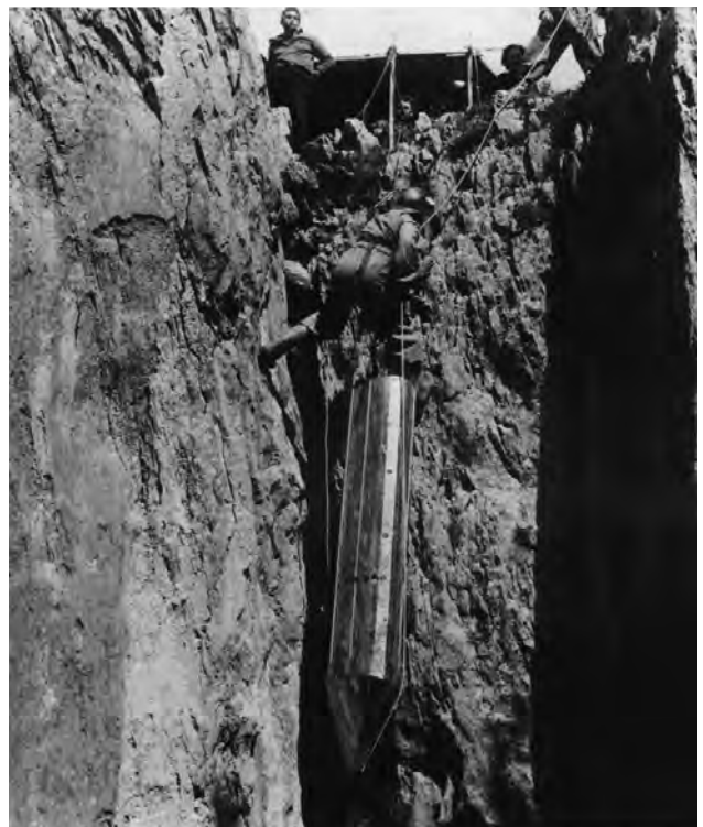
Figure 15. The container for Marcel Loubens' body descending the pothole.
