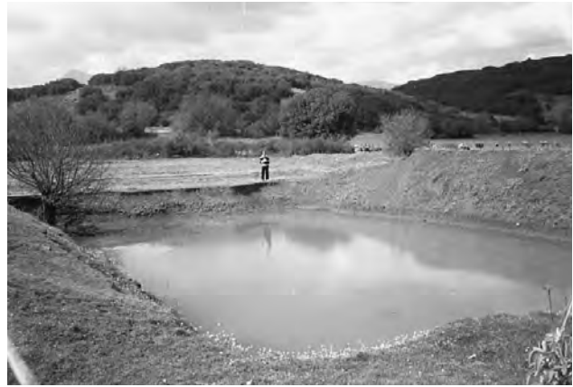
Figure 5. Excavated water reservoir about 10 m from Doline Fraksulis shown in Figure 4; water elevations differ based on supply and usage.
