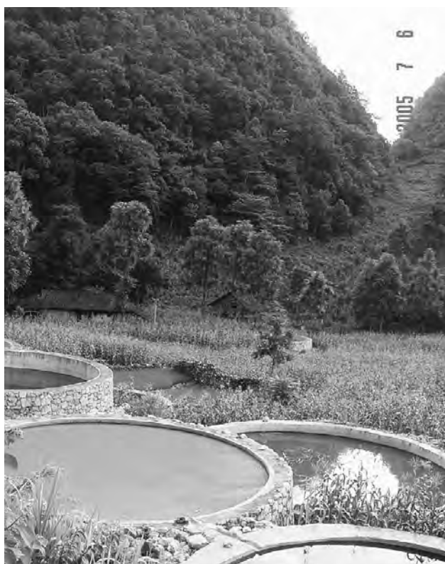
Figure 8. Water tanks harvesting rainfall, epikarst flow and overland flow in karst area, a piece of paddy field among corn is irrigated by the cellars.
