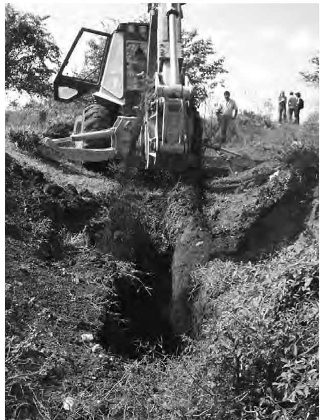
Figure 5. Backhoe excavating pit for geological examination.
