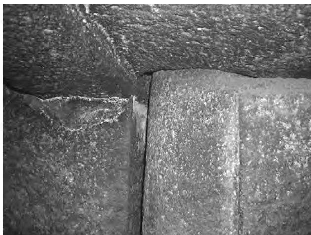
Figure 8. The door's lug fitted in the pit of the cover.
