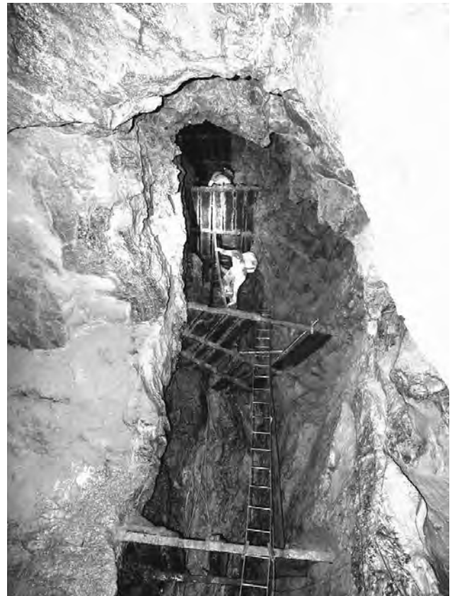
Figure 3. Wooden staircase in Grotta di Trebiciano, Trieste, Italy. These staircases have been initially installed in 1894 during the investigation for providing water for Trieste. The platforms (top in the photo) were installed one century ago in pitchpine treated with copper sulfate and carbonileo (Photo Maizan/SAS).
