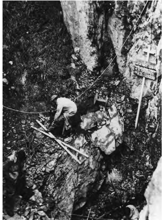
Figure 10. Assembling of the winch.
