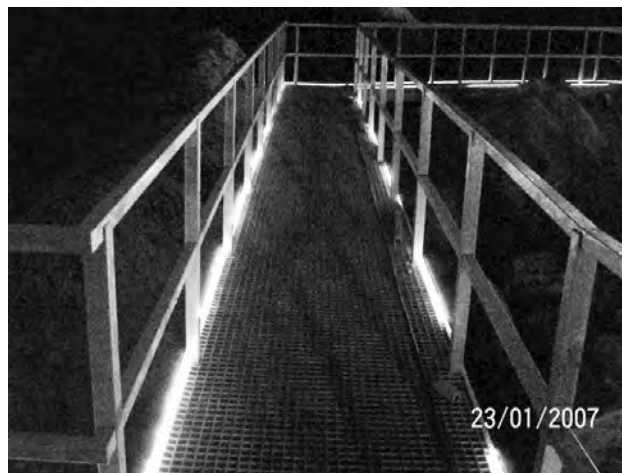
Figure 4. The emergency lights placed along the edge of the pathway in the Grutas de Bustamante, Mexico (Photo Cigna).
