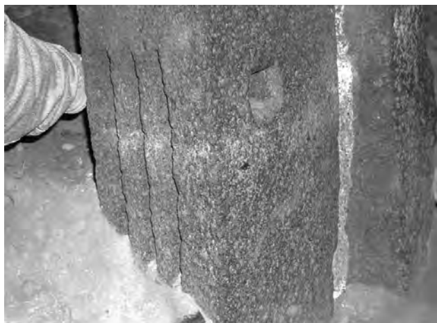
Figure 6. The stone doors are locked from inside with a lock. The lock can be made of a stone or wooden beam which passes through the rigid stone and enters deep into the pit over the door.
