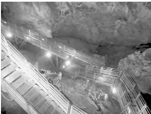
Figure 2. Zinc plated iron pathways in the Su Mannau Cave, Sardinia, Italy (Photo Cigna).
