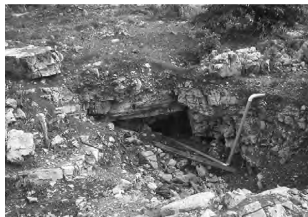
Figure 3. Sewage pipe into El Tragante; the cave entrance is 3 m deep.
