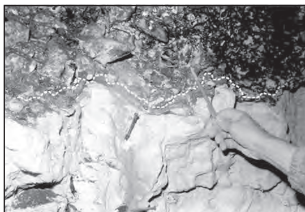
Figure 3: Contact between the overburden (CWF) and the chalk substratum (white). The dotted line delimits the hydrological screen consisting of compacted chalk alterites (photo. J. Rodet). One can distinguish the finely stratified structure in this impermeable layer of centimeter thickness.
