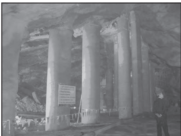
Figure 4: A big cave to be treated by ferroconcrete columns.
