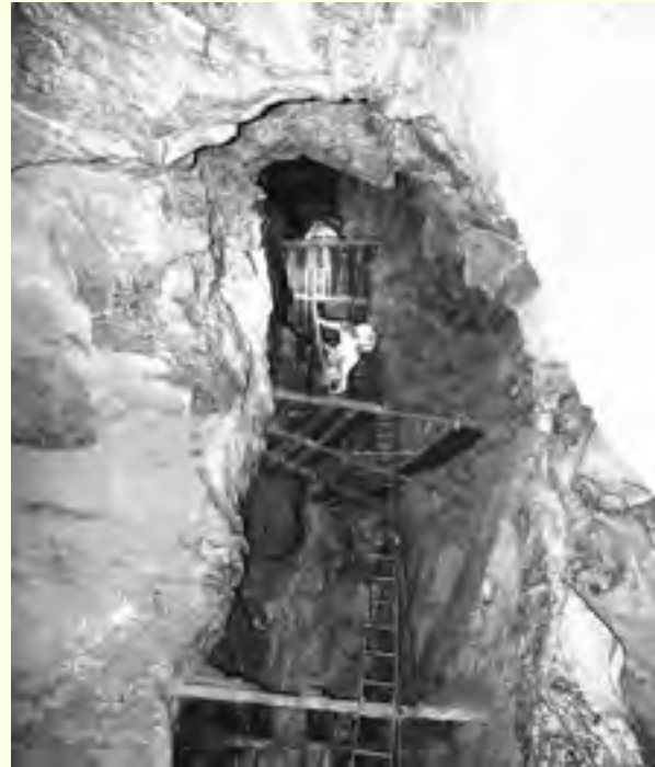
Figure 3. Wooden staircase in Grotta di Trebiciano, Trieste, Italy. These staircases have been initially installed in 1894 during the investigation for providing water for Trieste. The platforms (top in the photo) were installed one century ago in pitchpine treated with copper sulfate and carbonileo (Photo Maizan/SAS).
